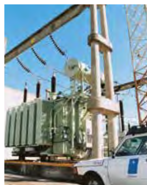
Rated Power 40 MVA. Rated Voltage 132 \pm 11 \times 1,427\% / 34,65 kV.
