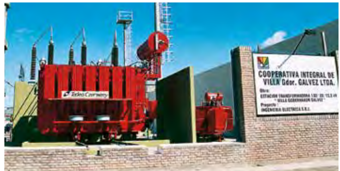
Rated Power 30 / 30 / 20 MVA Rated Voltage 132 \begin{matrix} +6 \times 1,67\% \\ -12 \times 1,67\% \end{matrix} / 34,5 \pm 2 \times 2,5\% / 13,86 kV. Earthing Transformer, 7640 kVA x 8 seg. / 5min., 13860 V.
