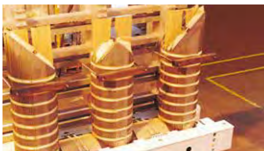
Transformer Core Rated Power 20 MVA
