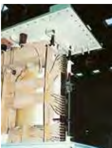
Auto Transformer Active Part Rated Power 30/30/20 MVA
