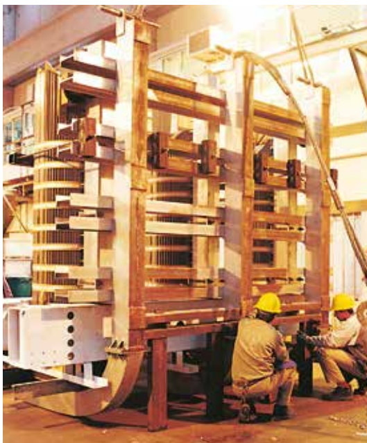
Transformer Core Rated Power 44 MVA
