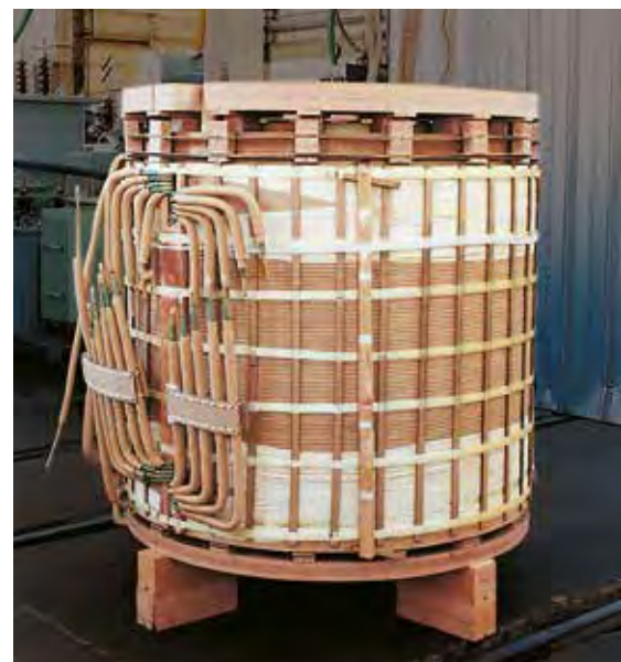
U Phase Leg Rated Power 40 MVA
