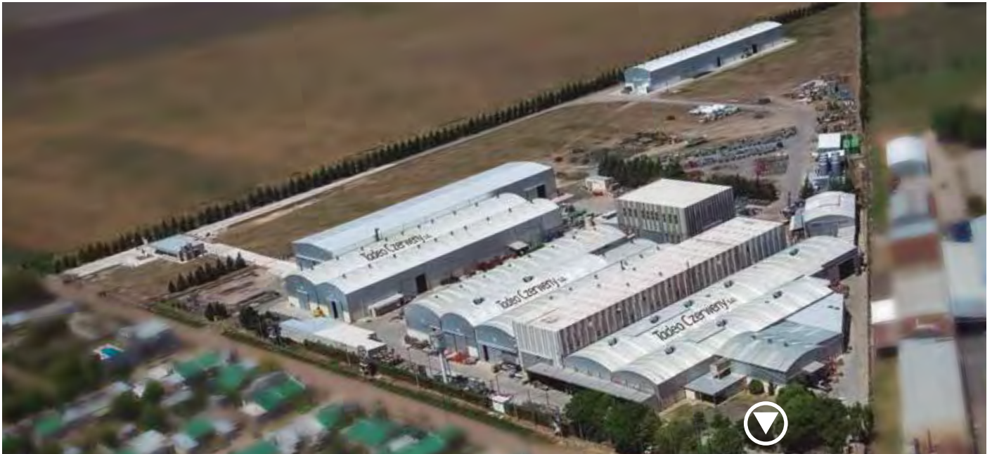
Industrial Plant view
