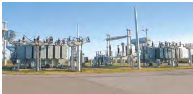
Rated Power 25/25/8,33 MVA Rated Voltage 132 \pm 10 \times 1,5\% / 34,5 / 13,86 kV.
